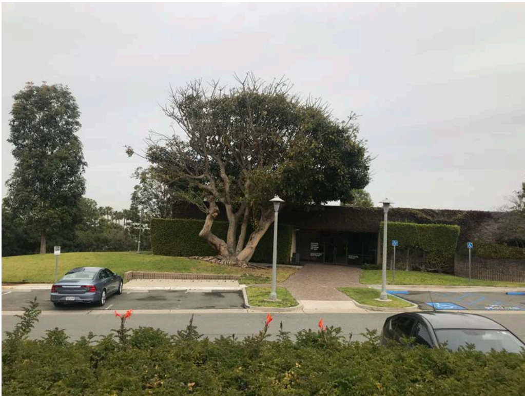
View of the subject property to the north 856 San Clemente Drive, Newport Beach, California
