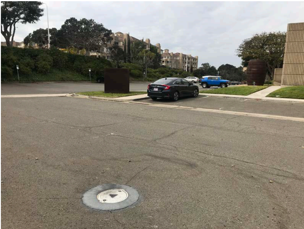
Groundwater monitoring well observed in the southeast corner of the property. 850 San Clemente Drive, Newport Beach, California
